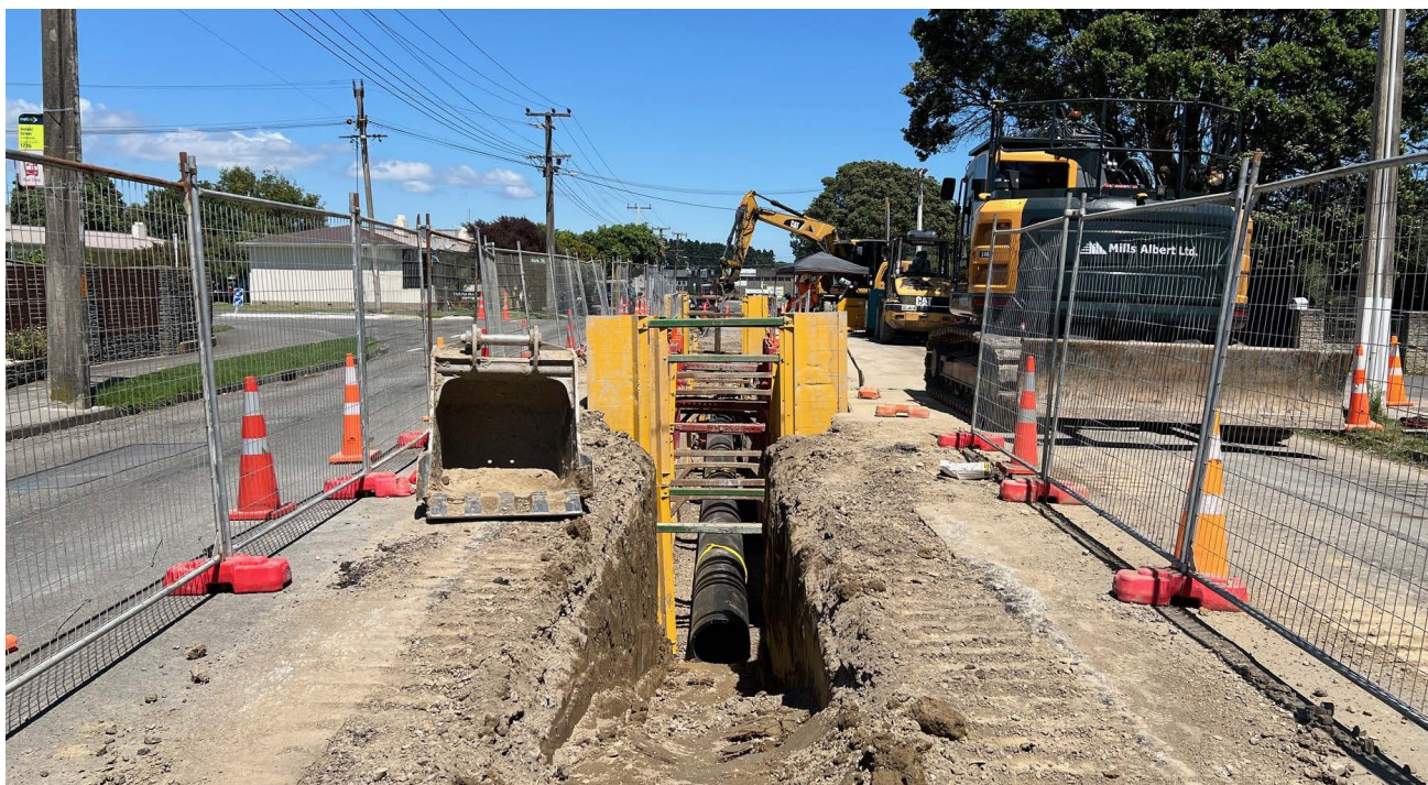
Installing new wastewater pipes along Mill Road and Aotaki Street, Ōtaki, as part of a major upgrade
