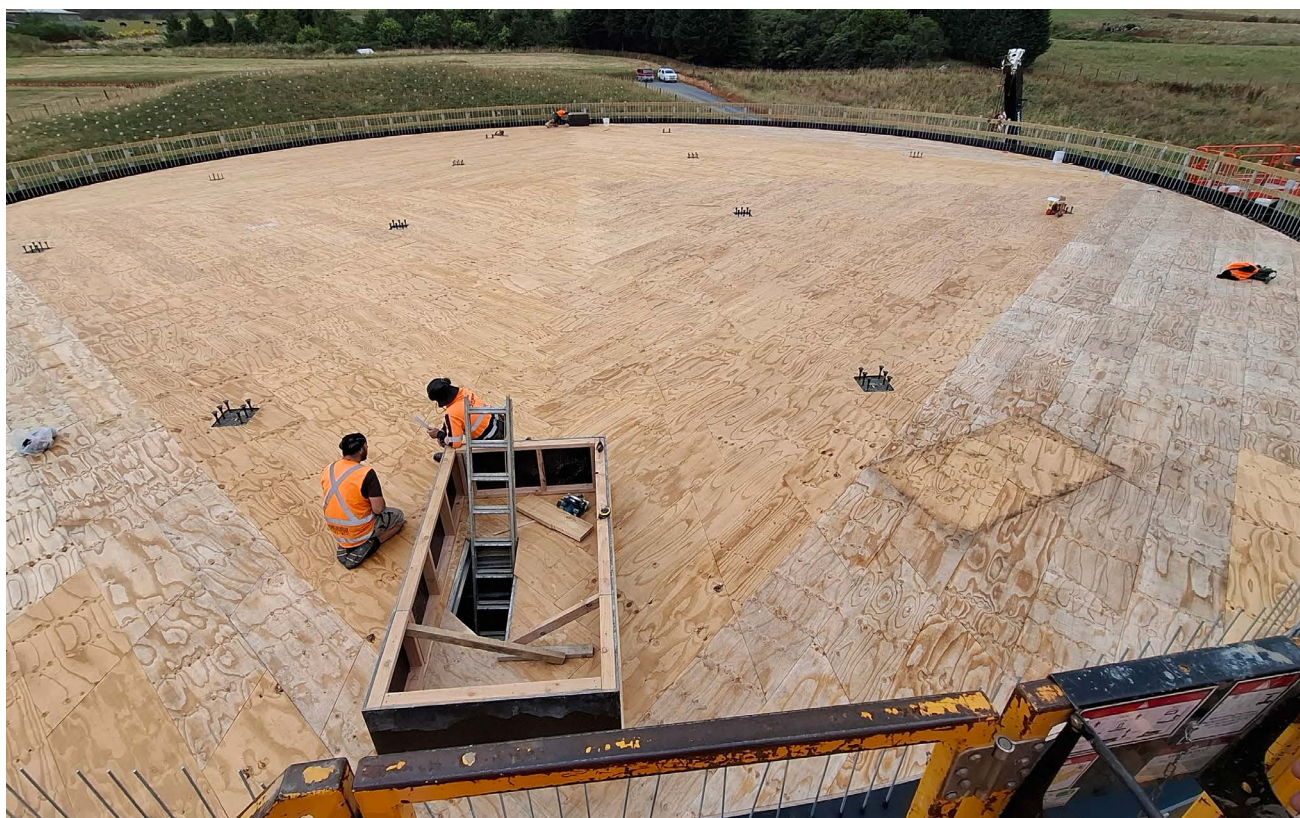
Formwork being installed at the new Ōtaki reservoir to prepare for the pouring of the concrete roof
