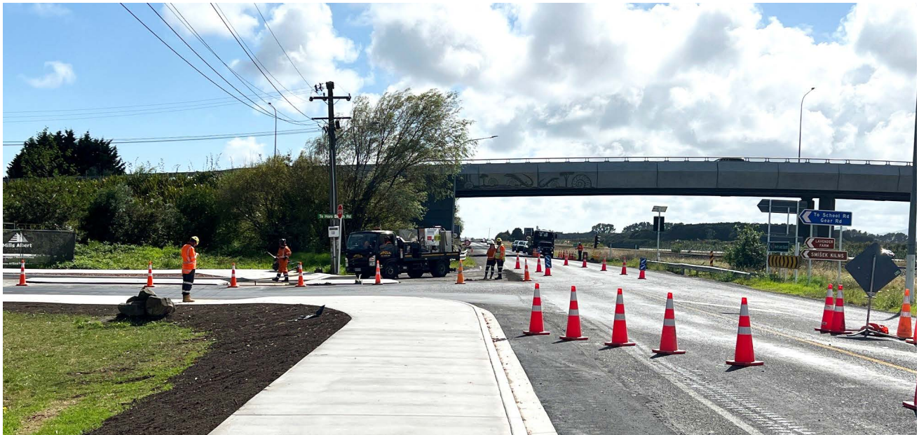
Work underway at the Te Horo intersection where the road is being resurfaced, and a new bus stop and kerb and channel are being installed.
