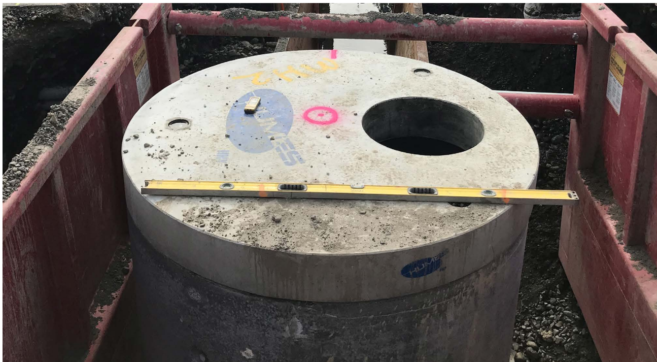
Installation of a manhole on Riverbank Road, Ōtaki
