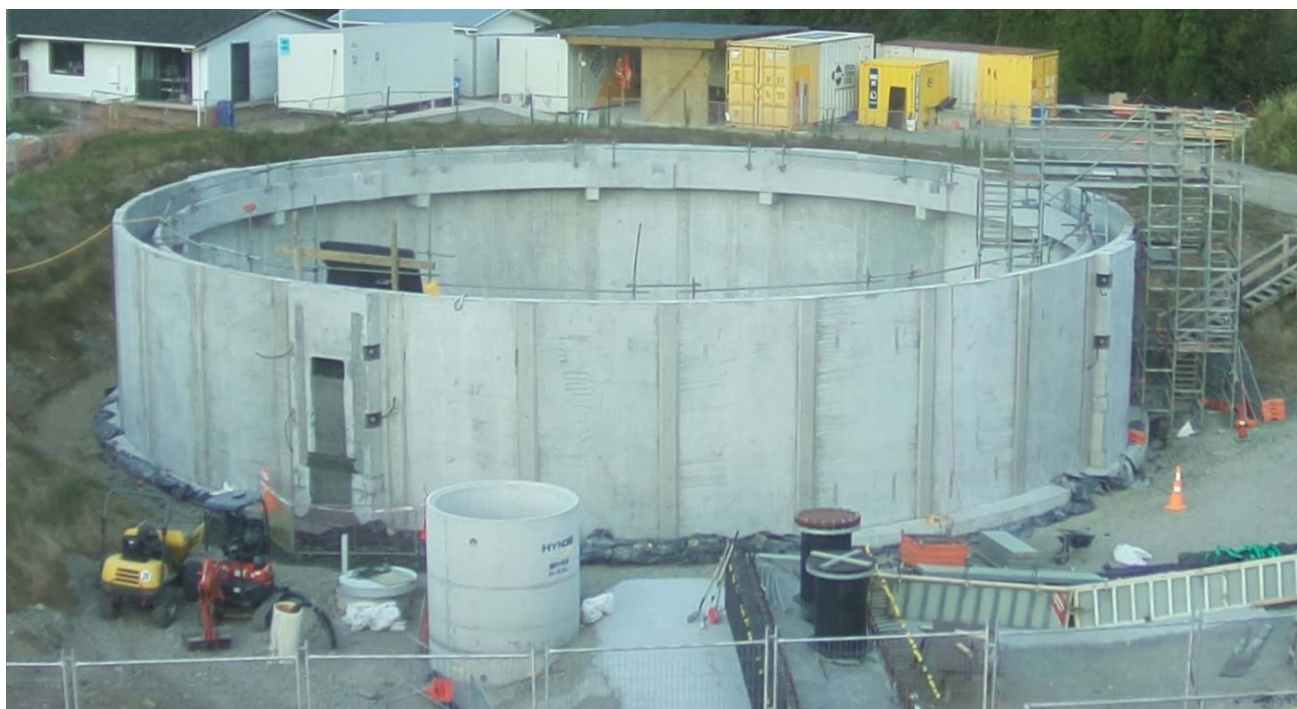
The new clarifier, a large tank which helps remove tiny particles from the river water, being built at Waikanae Water Treatment Plant
