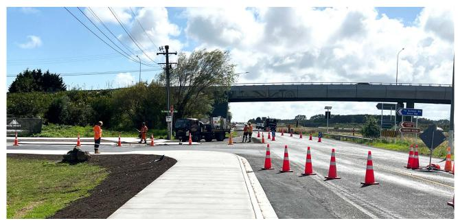
Work underway at the Te Horo intersection where the road is being resurfaced, and a new bus stop and kerb and channel are being installed.
