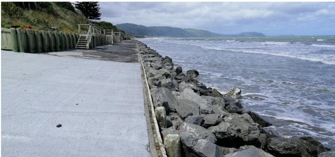
Figure 8.3: Old Coach Road in Raumati South, showing the toe rock riprap and the secondary timber wall behind it.
