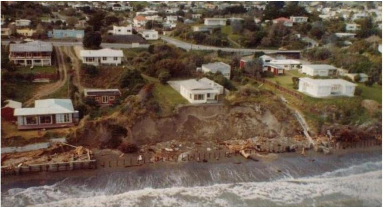
Figure 8.2: Coastal erosion behind failed coastal structures which fronted homes on Rosetta Road following the September 1976 storm (Image provided by KCDC).
