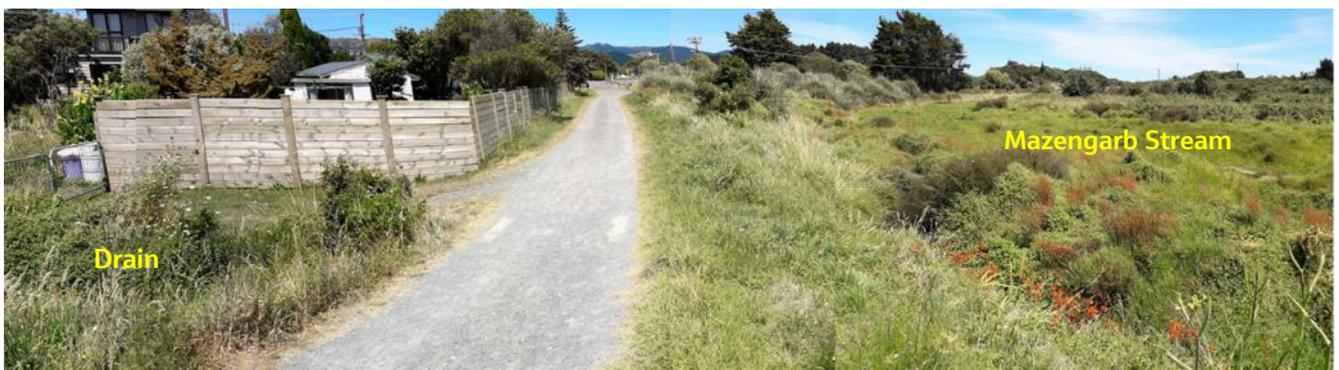
Figure 14.3: Otaihanga Boating Club access track off Makora Road. A culvert underneath the track provides an inundation pathway from the mouth of the Mazengarb Stream (to the right) to a stormwater drainage channel (to the left). The lowest levels on the access track are approximately 0.2 m below the present-day 1% AEP storm tide level.
