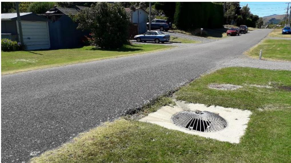
Figure 13.3: A "scruffy dome" inlet to the stormwater drainage pipe at the low point in Hemara Street. The pipe drains to the Waimeha Stream and water can flow back up the drain from the stream and out through inlets like this one when the stream water level is raised by storm tides. The ground level here is approximately 0.3 m above the present-day 1% AEP storm tide level.
