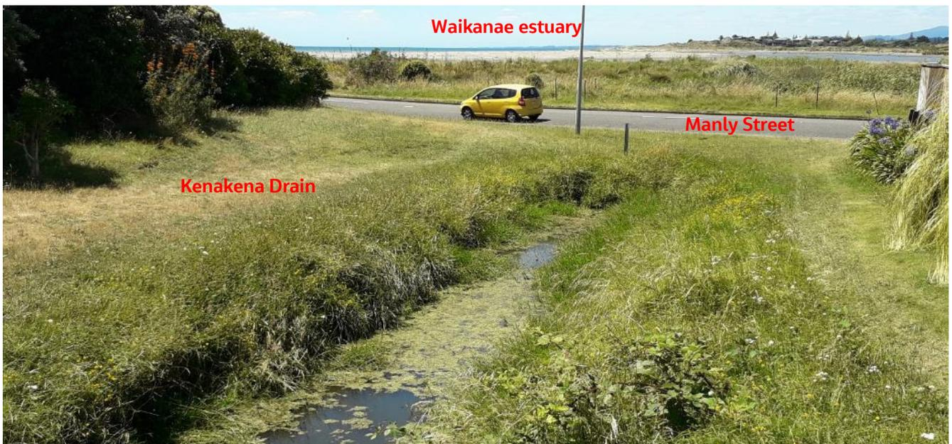
Figure 14.4: The Kenakena Drain is connected to the Waikanae estuary by a culvert under Manly Street and provides a pathway for coastal inundation both directly through the culvert and over Manly Street.
