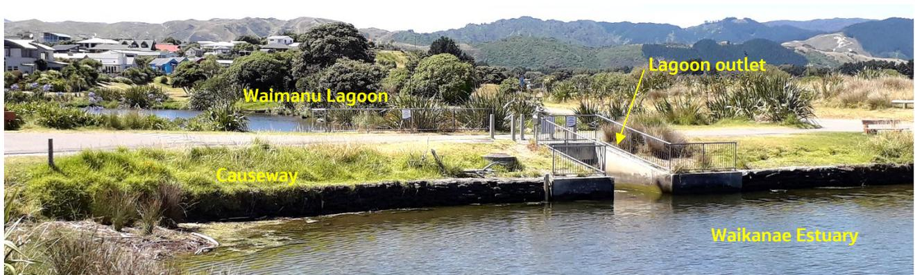
Figure 14.1: Causeway and outlet of the Waimanu Lagoon to the Waikanae Estuary. The road level on the causeway is approximately 0.1 m above the present-day 1% AEP storm tide level.
