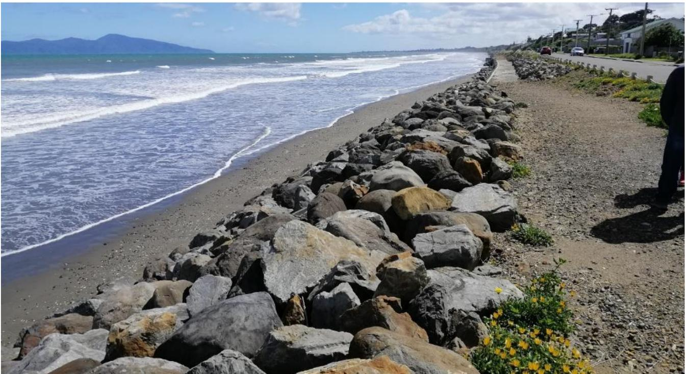
Figure 10.2: Rock revetment structure along The Parade, Paekākāriki.
