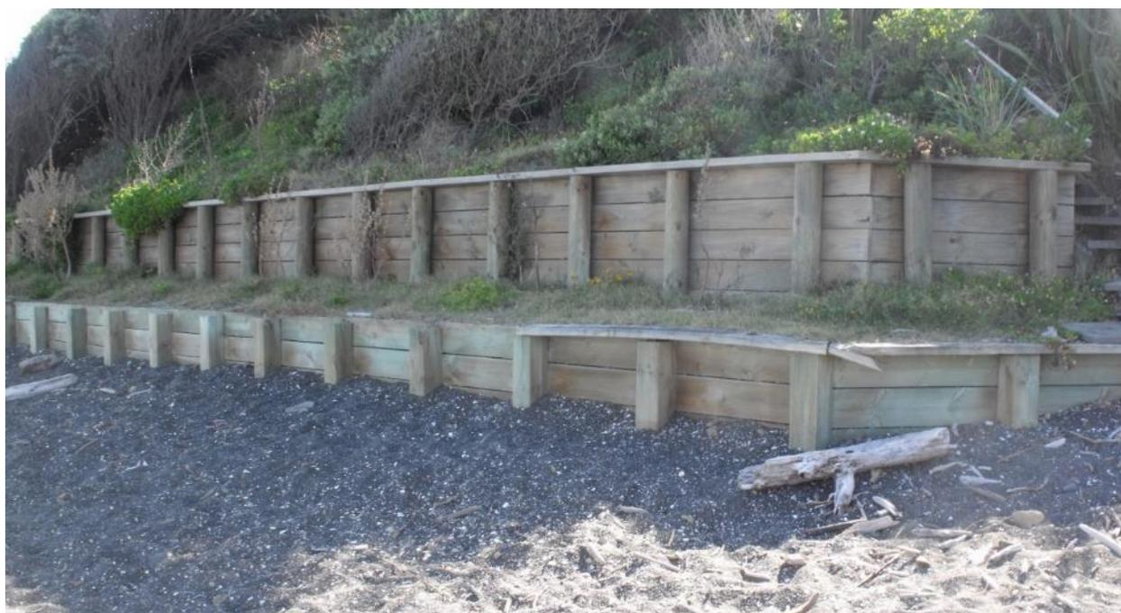
Figure 8.4: Private timber sea wall with primary and secondary structure (Image supplied by KCDC).
