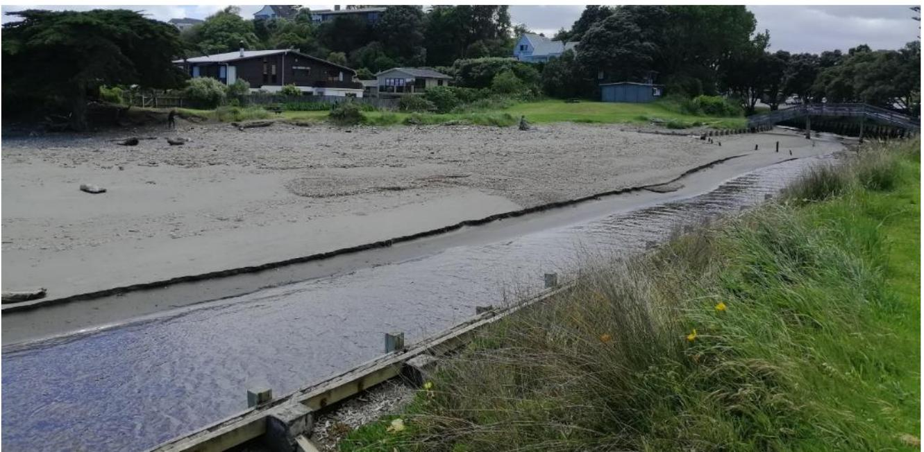
Figure 8.7: Wharemauku Stream facing upstream showing the timber training wall on the left bank of the stream.
