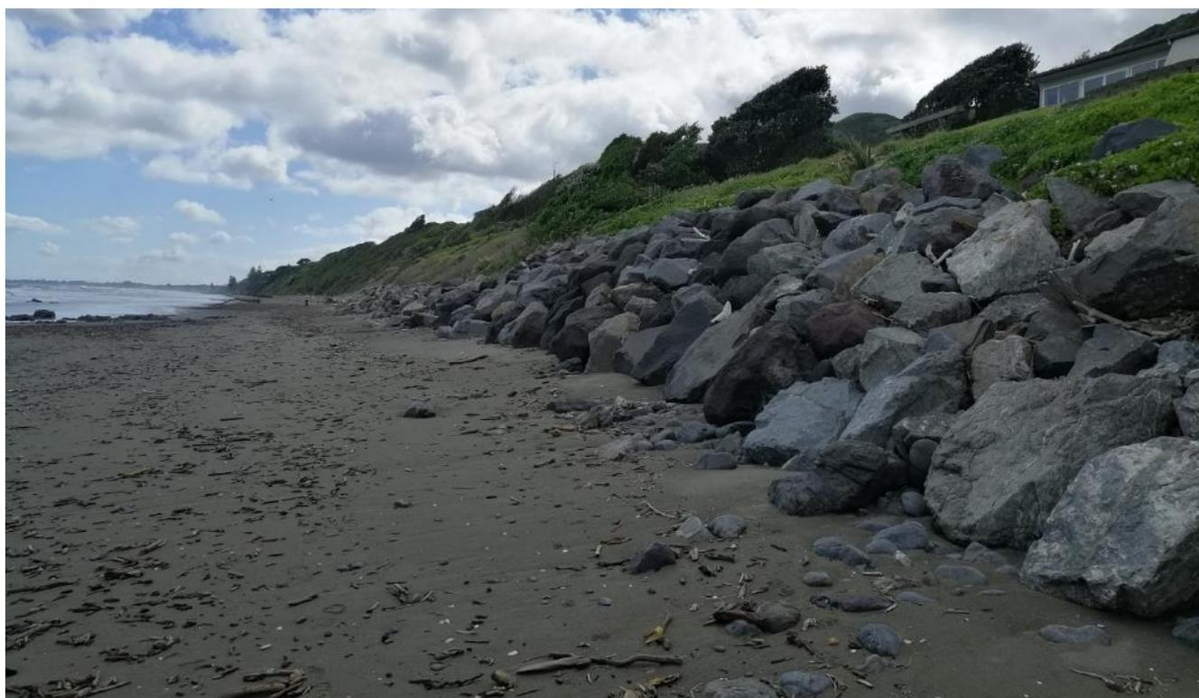
Figure 10.3: Rock revetment at southern end of Paekākāriki showing elevation of backshore.
