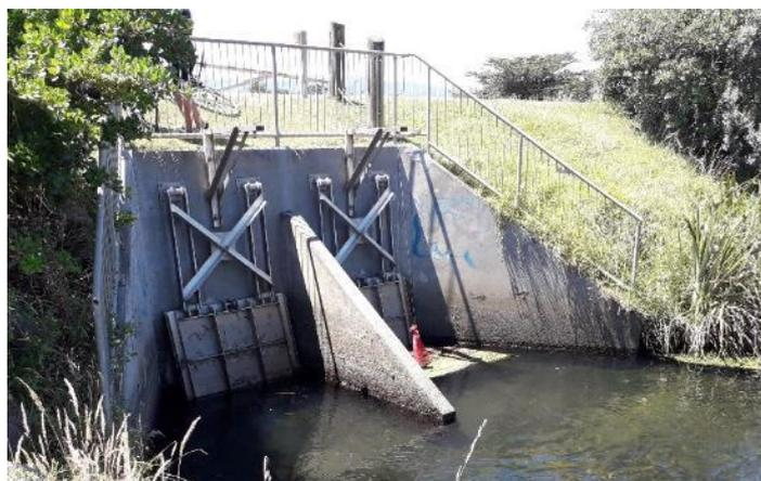
Figure 12.1: Floodgates on the outlet of the Rangiuuru Stream through the stopbank on the true right bank of the Ōtaki River mouth. The structure is viewed from the coastal side of the stopbank and shows the flap gates on the culverts which are pushed closed when the sea level rises above the water level in the stream on other side of the stopbank by the difference in water pressure.
