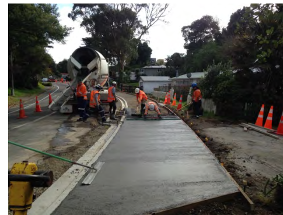
Poplar Avenue shared path under construction
