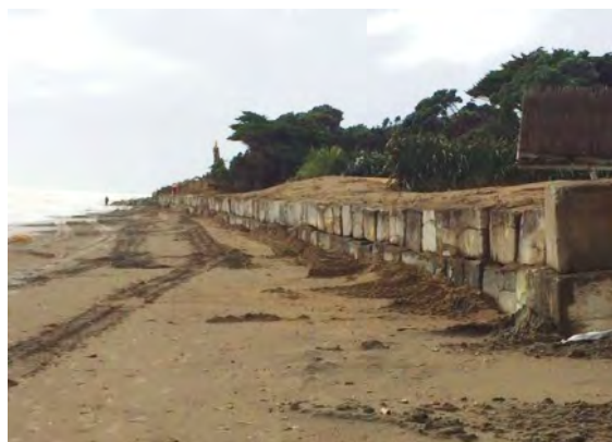
Wharemauku temporary block wall – built in three days following storm damage
