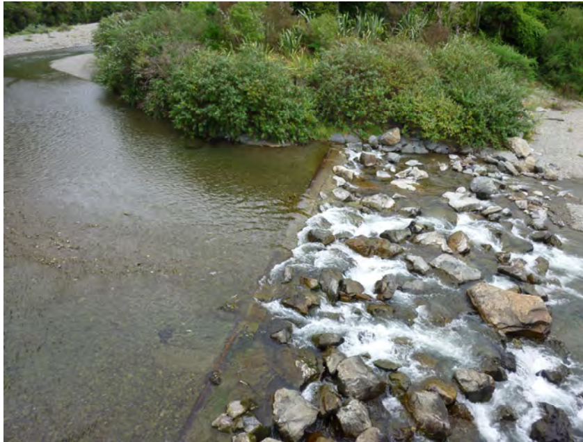
Figure 10-3: Existing Weir in Waikanae River at WTP
