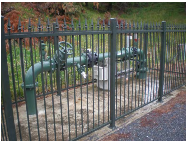
Figure 8-2: Existing Bore K4 Wellhead
