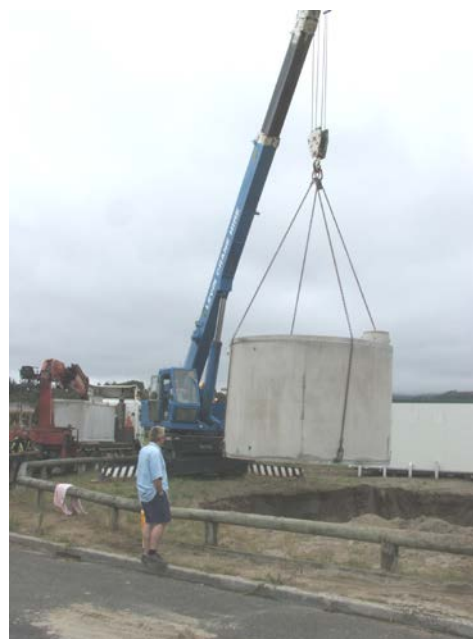
A 25,000 litre rainwater tank was installed at the Mazengarb soccer changing rooms to supply water for toilet flushing
