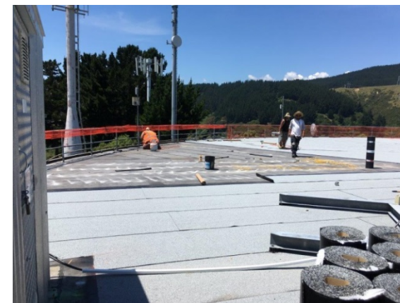
Application of a specialist coating to seal the roof of the Riwai water supply reservoir
