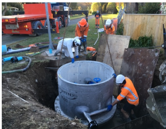
A new, pre-assembled valve chamber being installed at the Puriri Road wastewater pumping station
