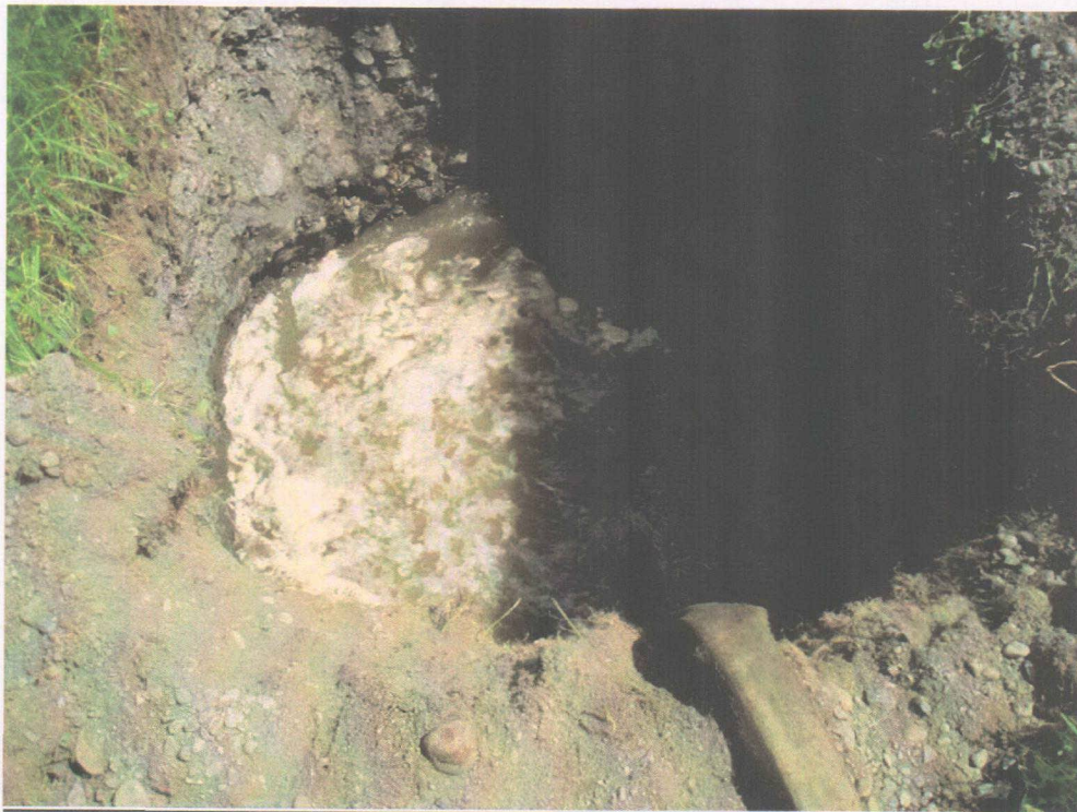
Excavation at start of test
