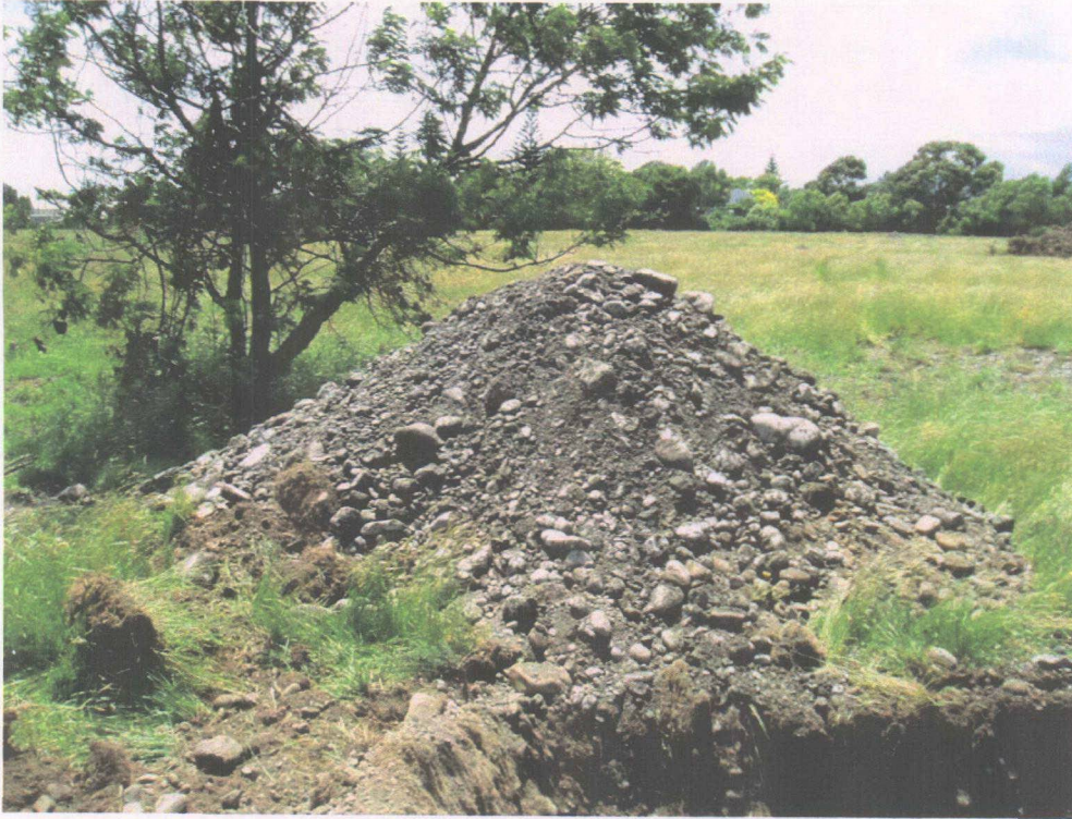
Typical excavated material stockpile
