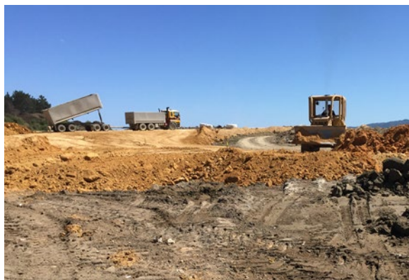
Final capping underway at the closed Otaihanga landfill
