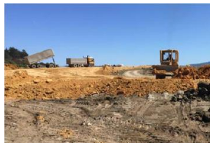
Final capping underway at the closed Otaihangā landfill
