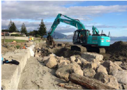
Realigning blocks and placing rock to strengthen the footing of the temporary Wharemauku block wall
