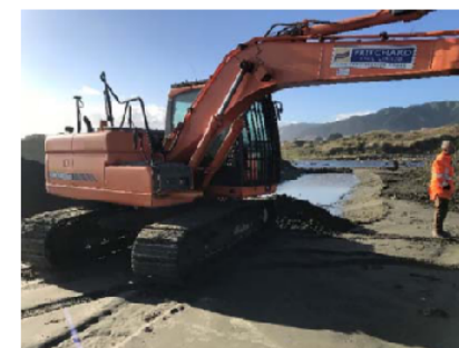
Stream mouth 'cutting' at Peka Peka in May 2019 to improve stream flow
