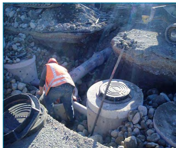
Installing stormwater pipes under a road
