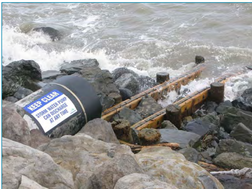
This pipe releases stormwater to the sea and carries a warning
