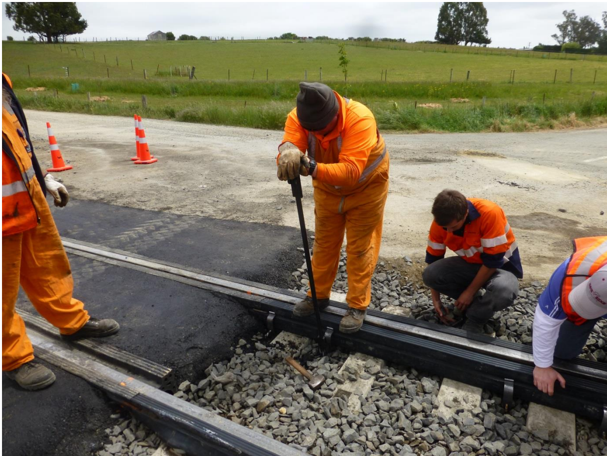
Figure 4: Example of the Polycorp Epflex Railseal Interface being Installed on a KiwiRail Level Crossing
