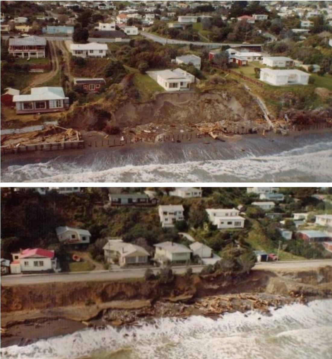
Figure 2.4: Coastal erosion behind failed coastal structures which fronted homes on Rosetta Road, Raumatī (top), and the Esplanade, Raumatī (bottom) following the September 1976 storm (Images provided by KCDC).
