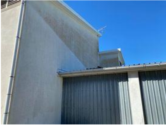
↑ Moss growing on monolithic plaster cladding
