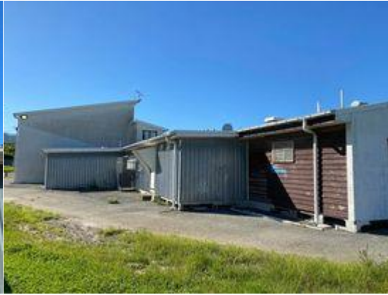
↑ Exterior iron cladding needs to be painted to stop it rusting.
