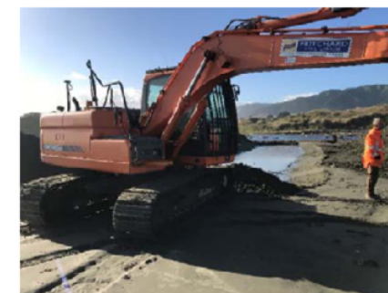
Stream mouth 'cutting' at Peka Peka in May 2019 to improve stream flow
