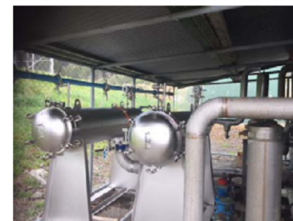
New micro-filters installed at the Paekākāriki water treatment plant
