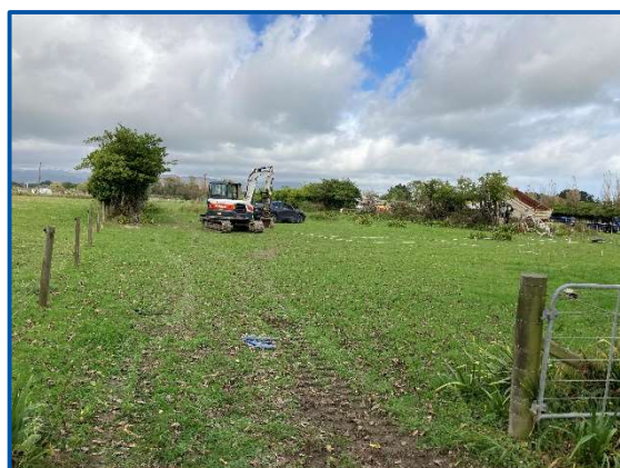
Photo 5: Looking south near the centre of the northern site boundary.
