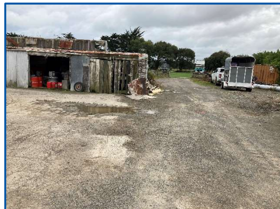
Photo 4: Looking north along the gravel access track. To the west of site a storage shed is noted with oil drums (red) noted. The shed is outside the site boundary.
