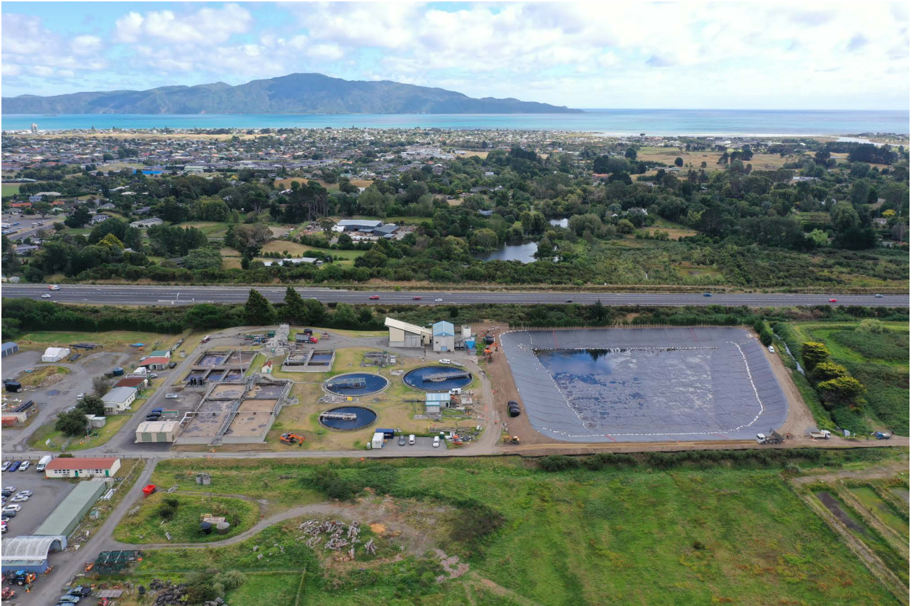
Paraparaumu wastewater treatment plant
