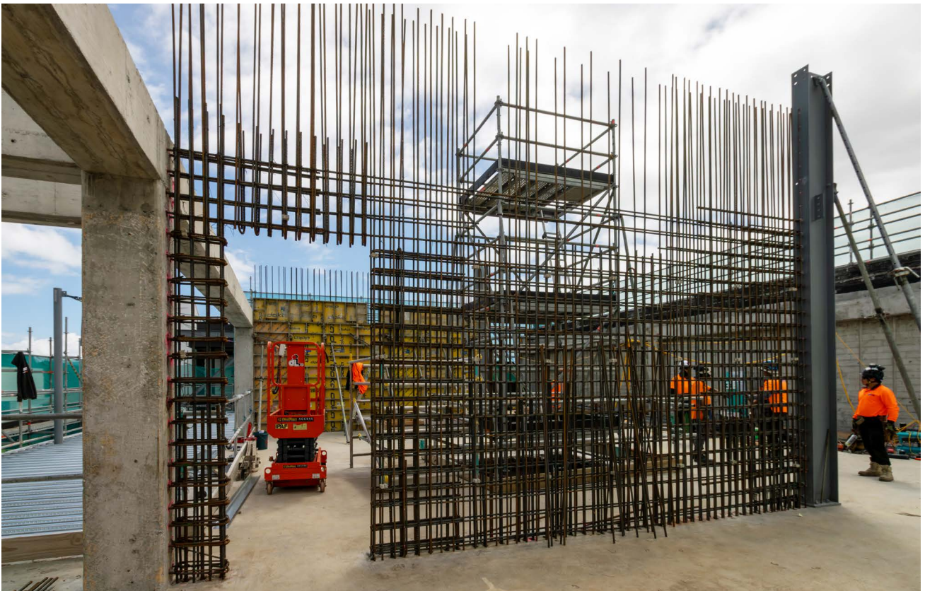
Te Ara Whetū (Waikanae Library and Hub) construction
