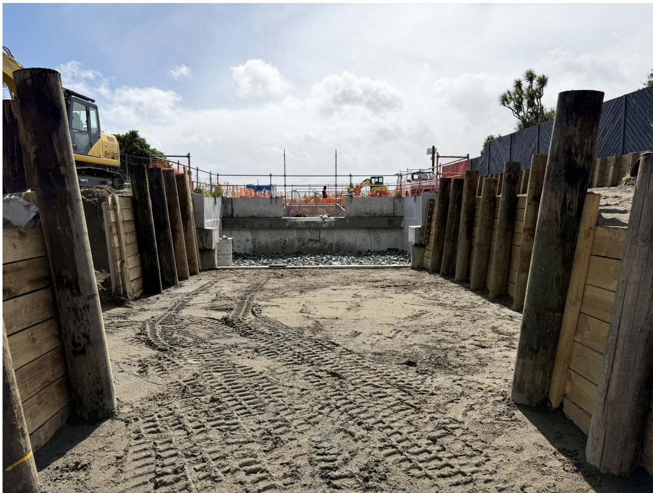
Construction of the Kenakena pump station
