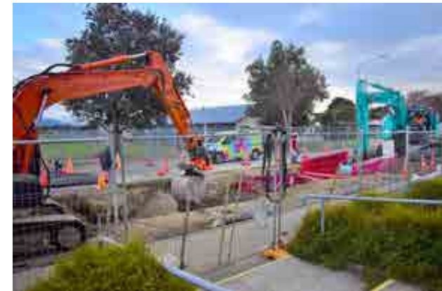
Amohia stormwater project.
