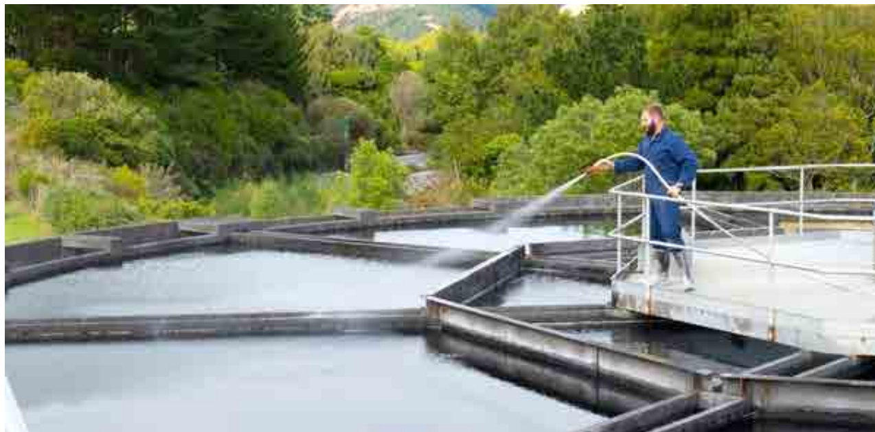
Hosing down the weirs of the Centra-floc Clarifier to remove organic build ups.
