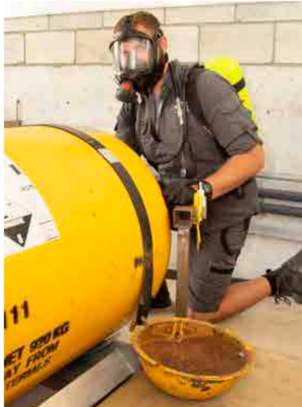
Replacing an empty 920kg 100% concentration chlorine gas cylinder.
