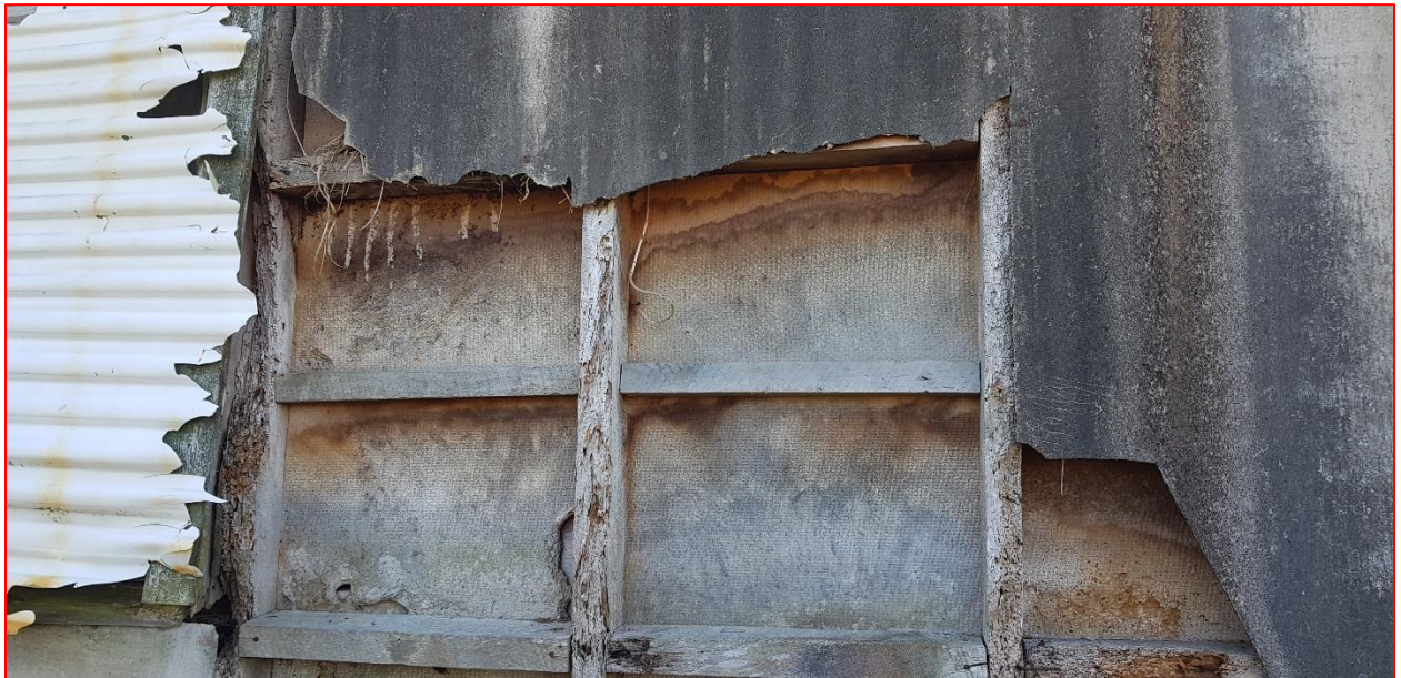
Photo 12: Damaged asbestos containing fibre cement sheet external wall cladding
