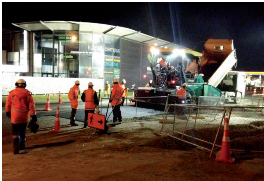
Night work on Kāpiti Road to reduce business disruption during opening hours.
