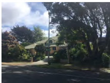
The precinct is characterised by deep front and rear yards with mature tall planting
