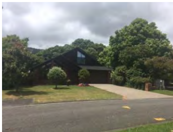
The precinct is characterised by a mix of one and two-storey buildings
