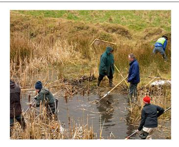
8.4.3 Accumulated sediments should be removed yearly or as need arises before the storage volume of the pond is threatened.
