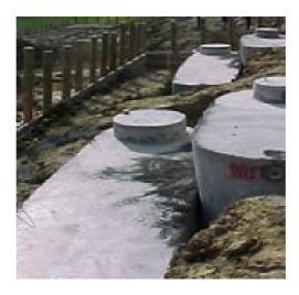
The tank may be above or below ground and is fed by site run-off, which usually includes a sump before the tank to intercept debris and coarse sediments. It generally has an inlet where water is fed into the top of the tank and restricted overflow outlet(s) connected to on-site disposal or public stormwater systems.
