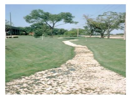
10.3.10 No vegetation or vegetation mulch shall be provided in the treatment filter bed surface. However, vegetative treatments include grass, mulches or shrubs may be used on the sloping areas of the basin outside the limits of the treatment filter. Mulches for shrubs on the slopes of the basin shall be non-bouyant materials.
